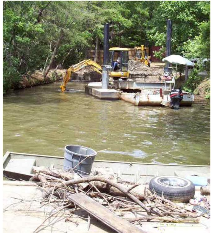
The dredger in action – along with a sample of trash hauled out of the lake. A poster on the barge indicated that debris removed from the lake in 2005 filled 161 large trash cans, 45 flat barge loads, and 14 harvester loads.
