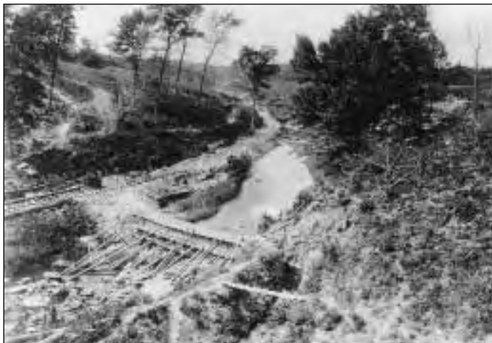
In 1913, the Piedmont Construction Company began building the Barcroft Dam by laying railroad tracks in the Holmes Run valley to transport rock for the dam and building a makeshift coffer dam to control stream flow. (September 13, 1913)
