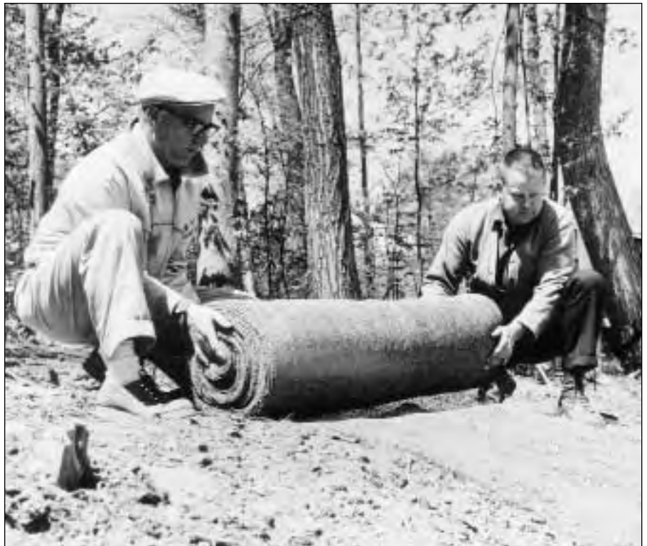
Marshall Augustine and Glen Anderson of the Soil Conservation Service of the U. S. Department of Agriculture install erosion control jute netting to a newly established demonstration planting at Beach 5. (June 1963)
