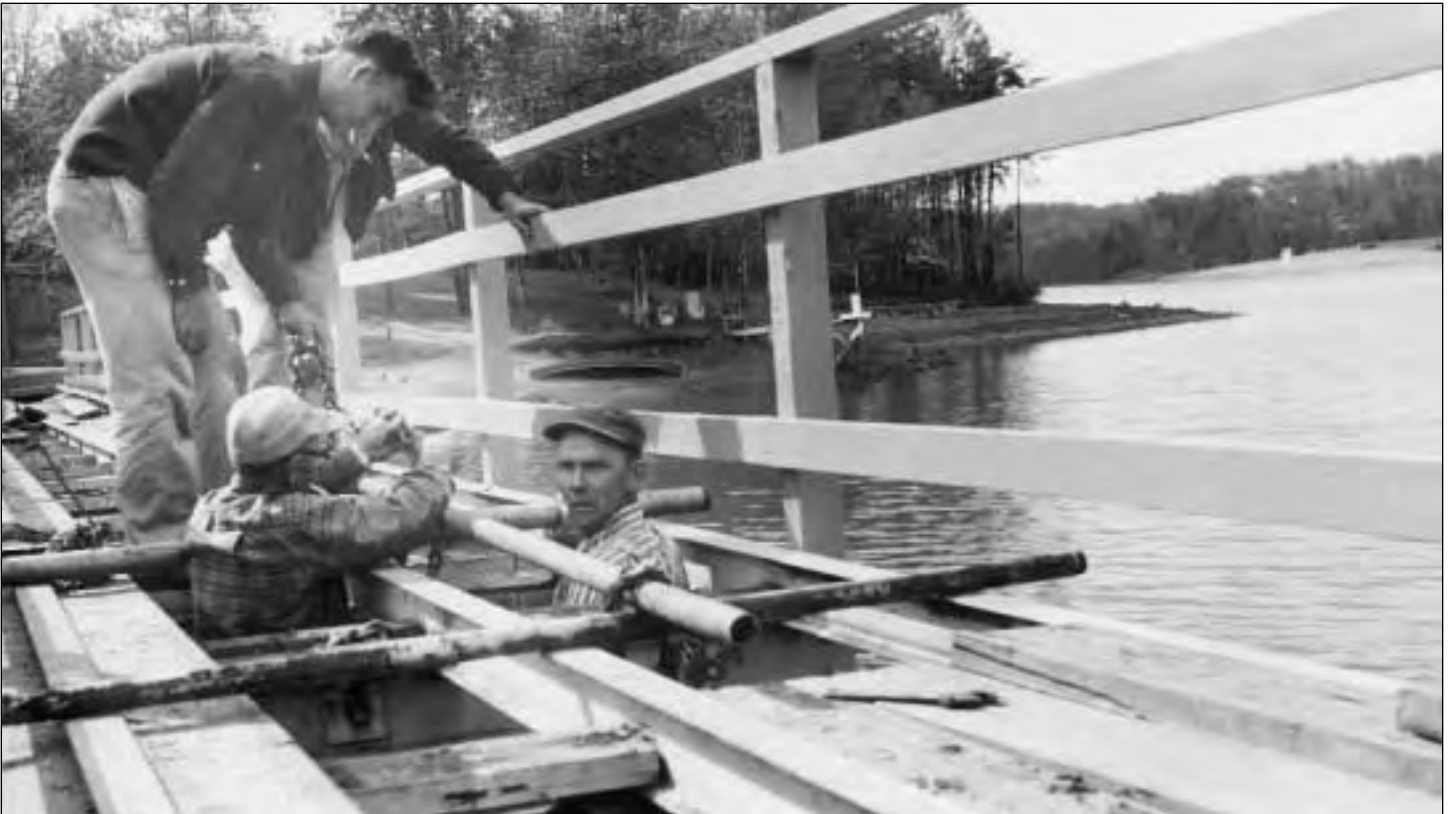
Four workmen are trying to figure out how to repair the decrepit old dam gates back in the 1960's. These wooden gates were supposed to open automatically during a storm, but usually they stuck. In fact, most of them stayed closed during Hurricane Agnes causing the failure of the Barcroft Dam and thus the creation of the Watershed Improvement District. (May 1963)
