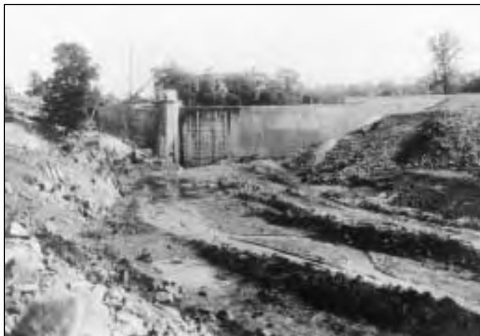
Completed, the Barcroft Dam supplied water to the City of Alexandria. Water company employees released water through underflow pipes. It flowed downstream and was recaptured at Duke Street in Alexandria and stored in a reservoir.
