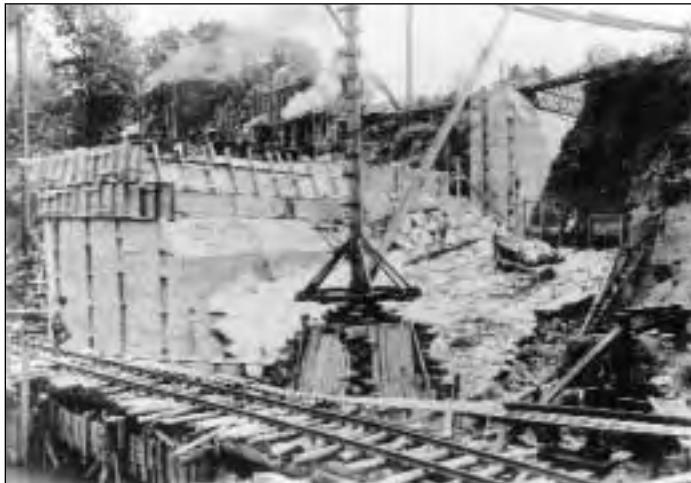
A rickety looking construction boom located by the railroad tracks unloaded large rocks to face the dam and partially fill its interior. The old quarry is now underwater off 3428 Mansfield Road in the North Area. (July 2, 1914)
