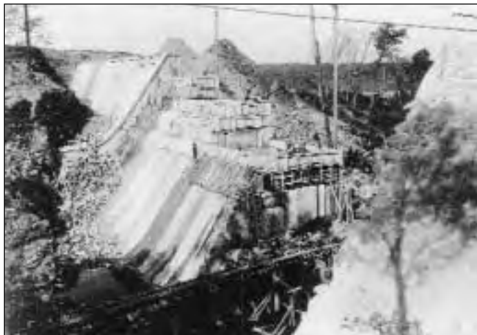
Lift by lift, the dam began to rise. With a gaping hole in the middle to accommodate the railroad tracks and to pass storm water, the two ends were constructed . . . slim at the far end, but fat in the middle to ensure stability. (November 2, 1914)
