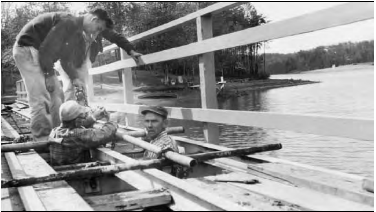
Four workmen are trying to figure out how to repair the decrepit old dam gates back in the 1960's. These wooden gates were supposed to open automatically during a storm, but usually they stuck. In fact, most of them stayed closed during Hurricane Agnes causing the failure of the Barcroft Dam and thus the creation of the Watershed Improvement District. (May 1963)
