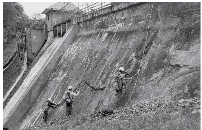
2012 —Erosion had taken a toll on the face of the dam. Workmen had to remove loose concrete from the east abutment.
