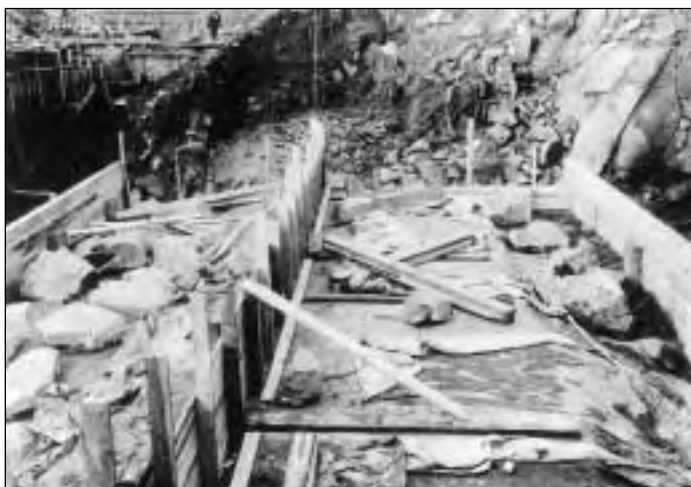
Engineers have quibbled whether the Barcroft Dam is a true Cyclopean Masonry structure. These rocks laid on top of concrete waiting for the next pour verify that it indeed does have a Cyclopean mix of rock and concrete. (November 30, 1913)
