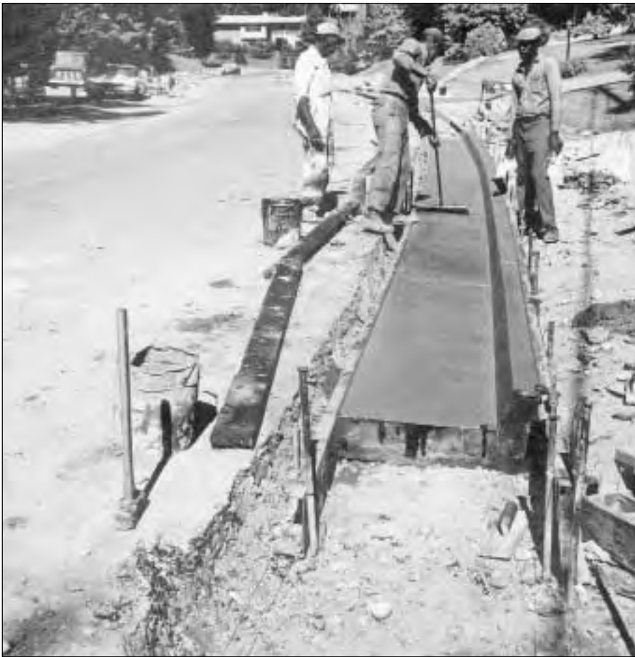
Responding to a WID engineering design by Ken Young of GKY & Associates, VDOT constructed a curb and gutter system to replace roadside ditches at the intersection of Nevius Street and Beachway Drive to improve safety of a school pedestrian crossing.
